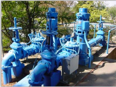
Storage Facility Rehabilitation
