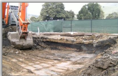
Soil Excavation in Phase 2 Area
