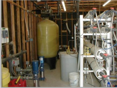
Existing RO domestic water treatment unit
