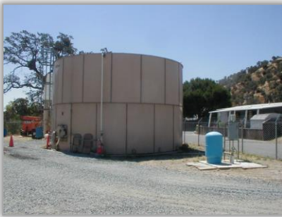
Domestic water supply tank and water supply well
