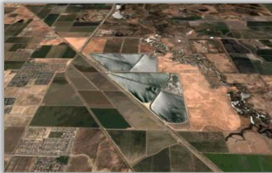
Aerial view of the City's facultative wastewater treatment ponds
