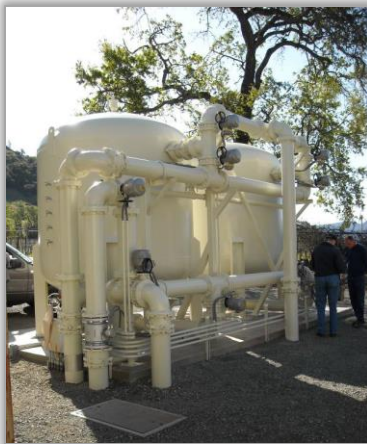
View of new pressure filter train added for redundancy and improved particulate removal
