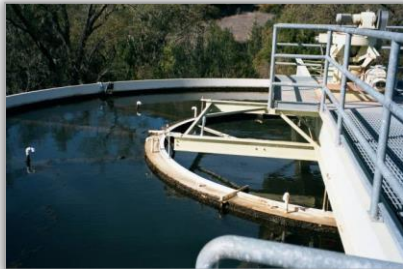
View of the primary clarifier to be modified as part of the project
