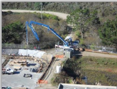
View of concrete placement for sludge drying bed retaining walls
