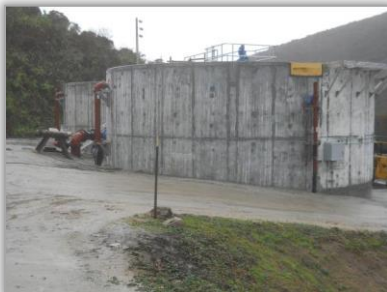
View of completed washwater recovery basins
