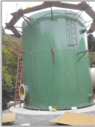
View of contact clarifier washwater supply tank in progress
