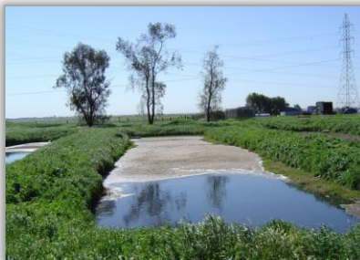
Anaerobic Treatment Lagoon
